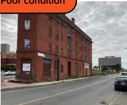
Flatiron Building, 533 Ann Uccello Street
